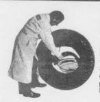
1. Remove flap inasmuch as it is not required on the drop center rim mounting and it prevents mounting the tire. Check to see tube is in casing and inflated sufficiently to prevent sag below tire beads.
