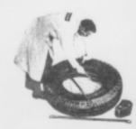
Lubricate last section of lower bead to facilitate mounting.
